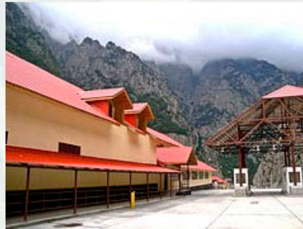
Border Crossing Station Kazbegi, Rep of Georgia
