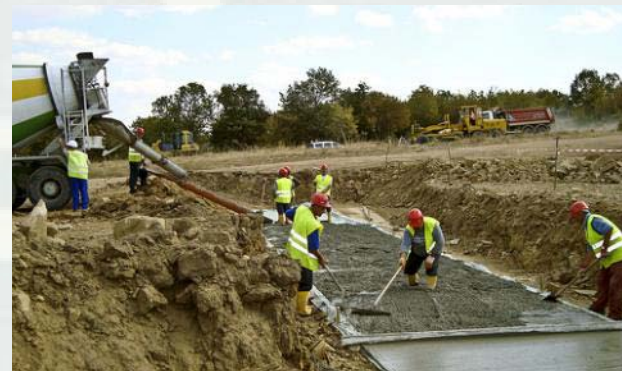
Construction at FOS Bulgaria Base Camp
