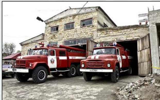
Comrat, Moldova On-going renovation of World War II-era converted fire station
